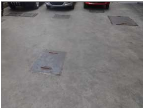
Underground Sewage Storage Pre-treatment
