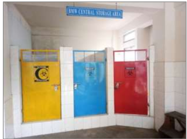
Biomedical Waste Main Storage
